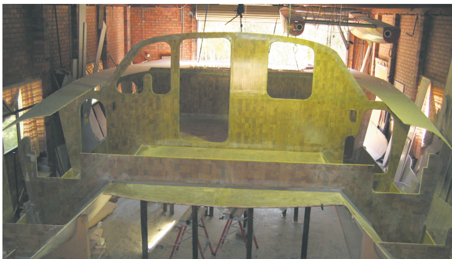
Assembly underway, main bulkheads, chamfer panels and bridgedeck installed. (above) Deck moulds with two decks just released. (below)
