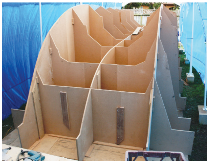
MDF Build frame assembled.
